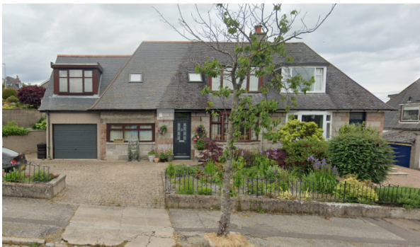
43 Morningside Avenue- no records available
