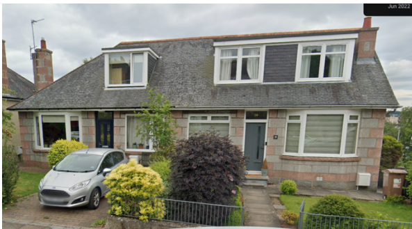
39 Morningside Avenue- no records available
