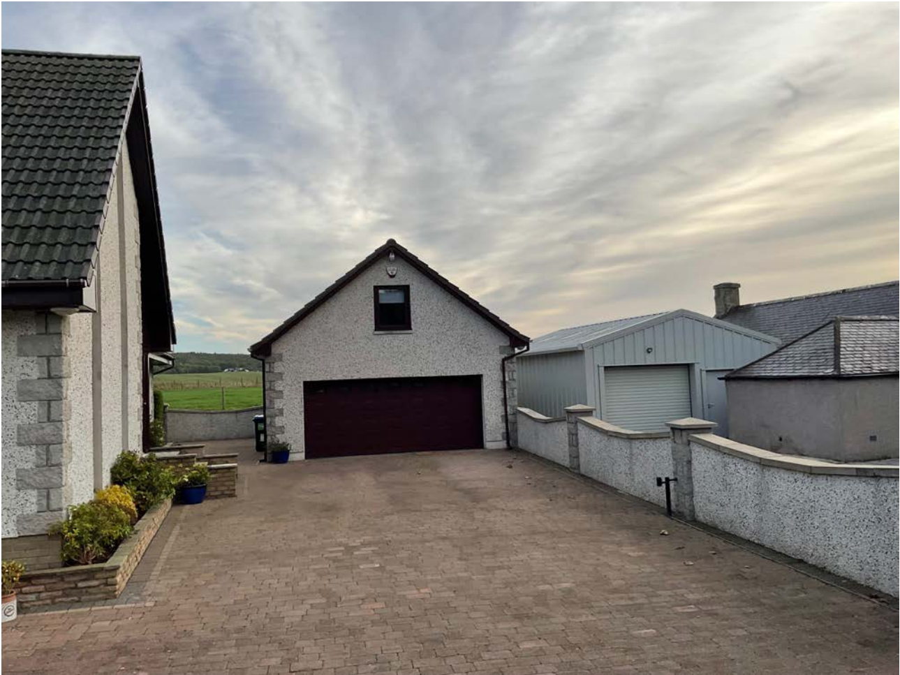
Fig 3 Applicants Garage to the left, Steel Garage to be re-cycled centre and cottages to the right of photo.
